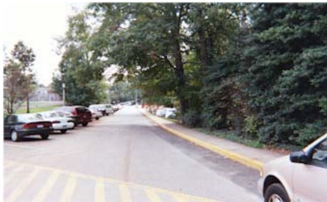
(Clockwise from top left) Infiltration Trench is on downhill side of roadway; Infiltration Trench is installed; Infiltration Trench is paved with standard pavement material
